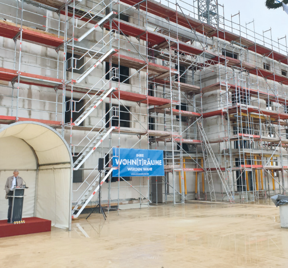
Richtfest in Reeshoop, Ahrensburg
